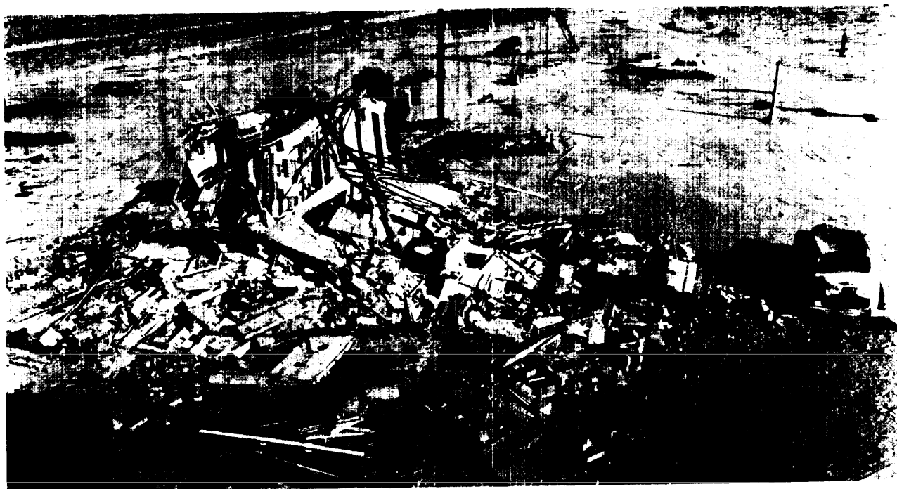
Damage to unreinforced brick house (5-psi overpressure)
